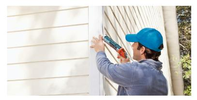
NovaFlex Multi-Purpose Adhesive Sealant is a premium all-weather medium modulus silicone that stays flexible and is resistant to cracking and discoloration. The cured sealant resists mildew. This premium allweather silicone is tack free in 10 minutes and is completely cured in up to 2 days.
